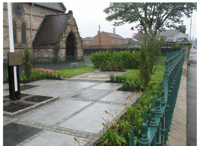
St. Mary's Church after the refurbishment work
